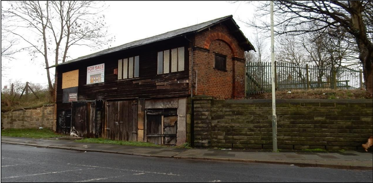
Plate 13. The Lime Depot. Waggon's approached the building along the branch line from the left (at a high level), passed through and dropped their loads through trap doors in the floor where the lime fell into bays. Builders could then purchase and collect lime from the ground floor level where carts could back up to the bays and then head back to where the lime was needed.
