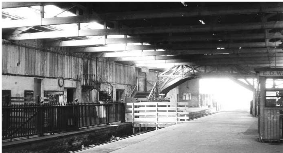
Plate 6. The station interior, looking west, in the early 1970's. By then North Road had been reduced to a halt. We see the wooden footbridge which the NER provided after linking through the two bays to provide another through line; BR had no need of this second line and therefore substituted level access. The footbridge and the kiosk on the right still feature in the present museum 20 as does the clock, the spiral staircase and the railings.
