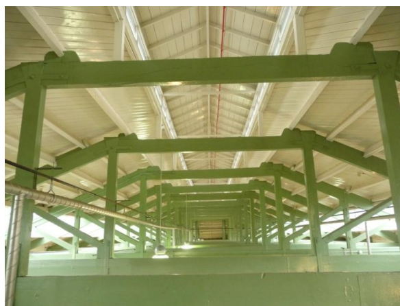
Plate 25. The original 1842 Queen post trusses
