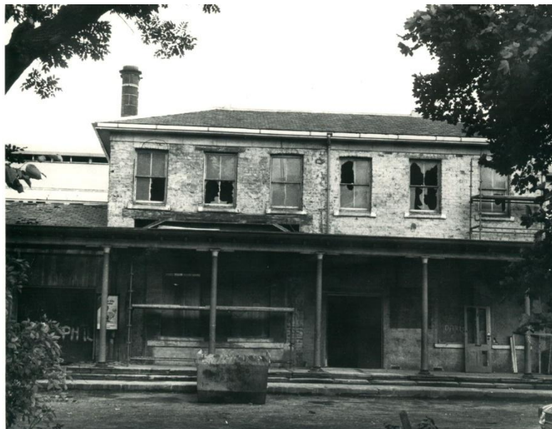
Plate 8. The front elevation during restoration works 1973-4. The upper floors are of brick but the lower ones appear to have been patched in brick, but may have been sandstone rubble originally (photo: courtesy of the Centre for Local Studies at Darlington Library 1761a)
