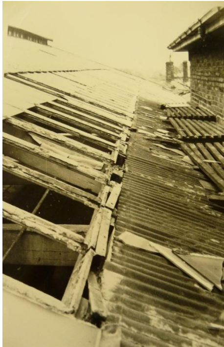
Plate 26. The train shed roof at the join with the upper storey of the station before restoration
