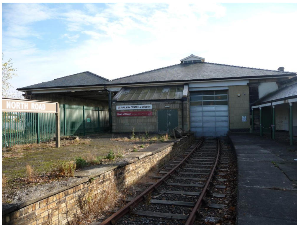
Plate 18. The same view in 2014. The platforms are intact, the renewed shed roofs appear to be in good condition, but the blocking to the train shed has lost any visual permeability that the original train shed had
