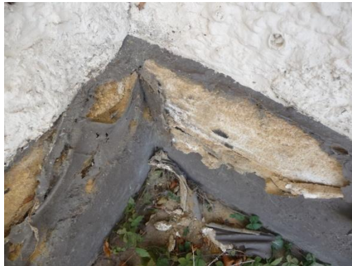
Plate 15. Paint is peeling off the sandstone stylobate and the stone is disintegrating beneath
