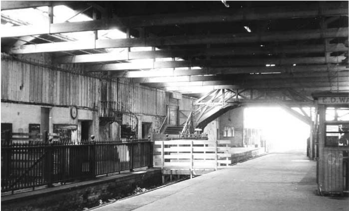
Plate 22. Train shed interior with the north elevation on the left looking towards the ticket office entrance and clock and spiral staircase dating to 1876 when the upper floor was added. The upper floor appears to be clad in timber.
