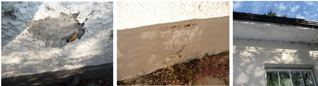
Plate 10. Left: Cracks in cementitious render are caused by lack of breathable materials and lack of maintenance. Such damage leads to damp internally and damage to stone or brickwork beneath. Centre: non breathable paintwork and cementitious coatings to the stylobate have resulted in decaying stonework behind. In this instance an air vent has also been cemented over. Right: vegetation is growing out of gutters which needs to be cleared before resulting in expensive damage and further water ingress
