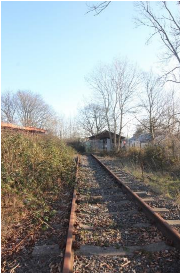
Figure 67. The Darlington branch line today bypassing the lime depot in the distance which had its own spur carrying waggons into the depot
