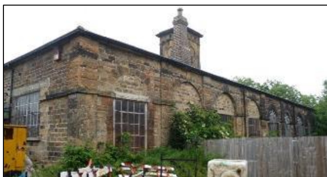
Figure 78. The south elevation of the Goods Shed 2012
