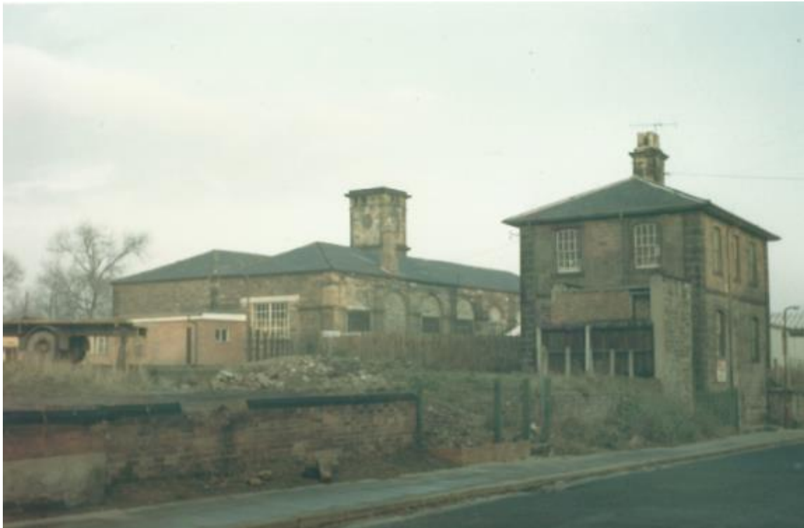
Figure 48. The close relationship between the Goods' Agents' Offices and the Goods Shed can be seen in this photo from 1970. There had previously been an S&DR building in the vacant plot left of the offices (photo: John Proud Collection, courtesy of Win Proud)
