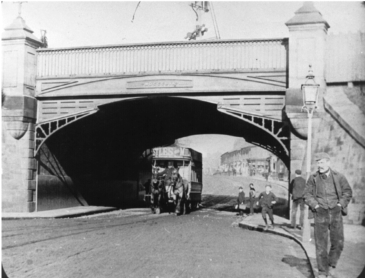
Figure 35. This photo pre-dates the replacement parapets that are there today; some additional fretwork has been added since the Network Rail plans were drawn above.
