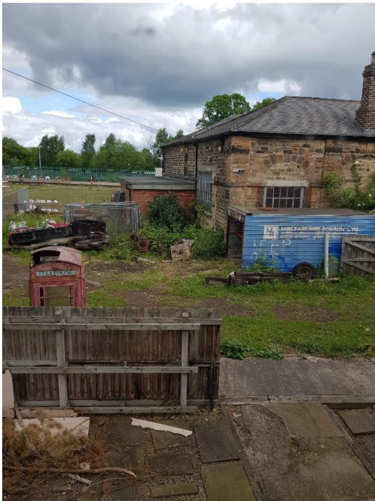
Figure 55. The Goods Shed as seen from upstairs in the Goods' Agents' Offices – a building currently difficult to appreciate but due a new lease of life before 2025
