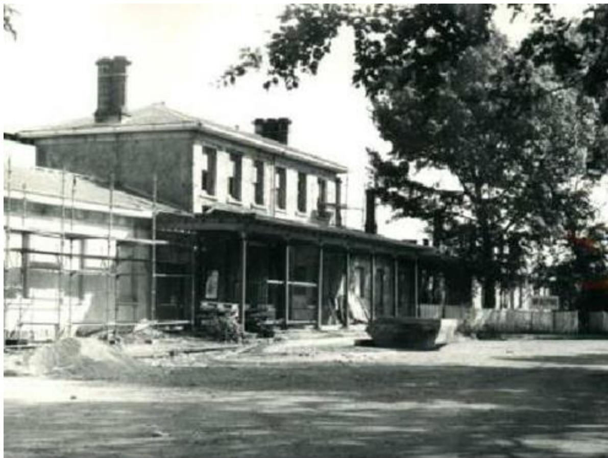
Figure 43. The station during restoration works in 1975 (photo source unknown)
