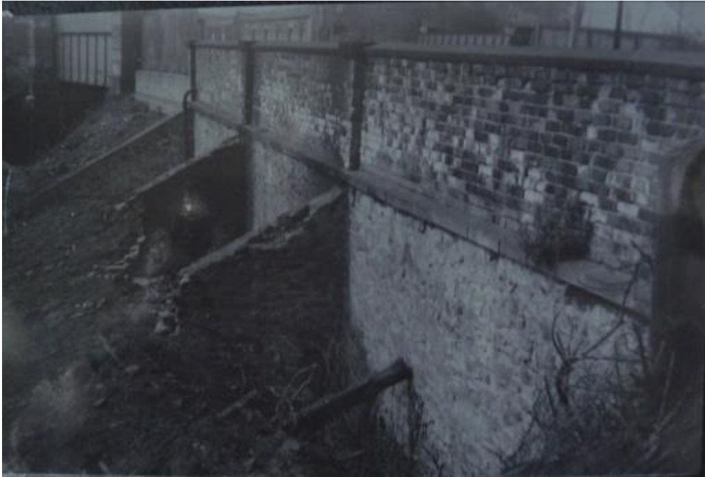
Figure 74. The site of the former Merchandising Station. The railway embankment has either had buttresses added or these are the remains of the station walls which separated each unit/cottage. The latter interpretation seems most likely because their uneven size matches early depictions of the station. The photo is undated but is possibly late 1960s/ early 1970s. Photo: John Proud Collection, courtesy of Win Proud.
