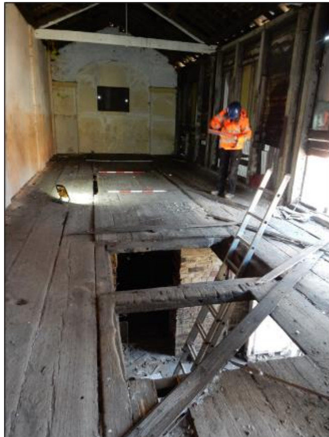
Figure 26. View along the upper floor looking SE. Original timberwork survives to the left and right of the modern openings and formed platforms where attendants could stand to operate the waggons' bottom-opening doors and deposit the lime into the cells below. The narrower central planks are all later insertions to block the gap between the waybeams. The ranging poles mark the positions of two of the ground-floor walls that divide the cells below (photo: Archaeo-Environment Ltd).
