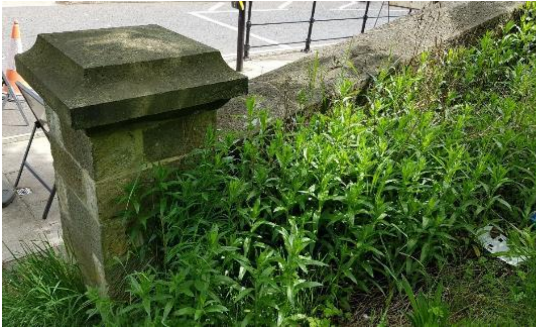
Figure 19. The surviving gatepost built into the boundary wall on Bonomi Way.
