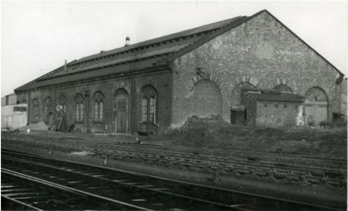
Figure 37. The engine shed's west elevation. Photo: Ken Hoole Collection
