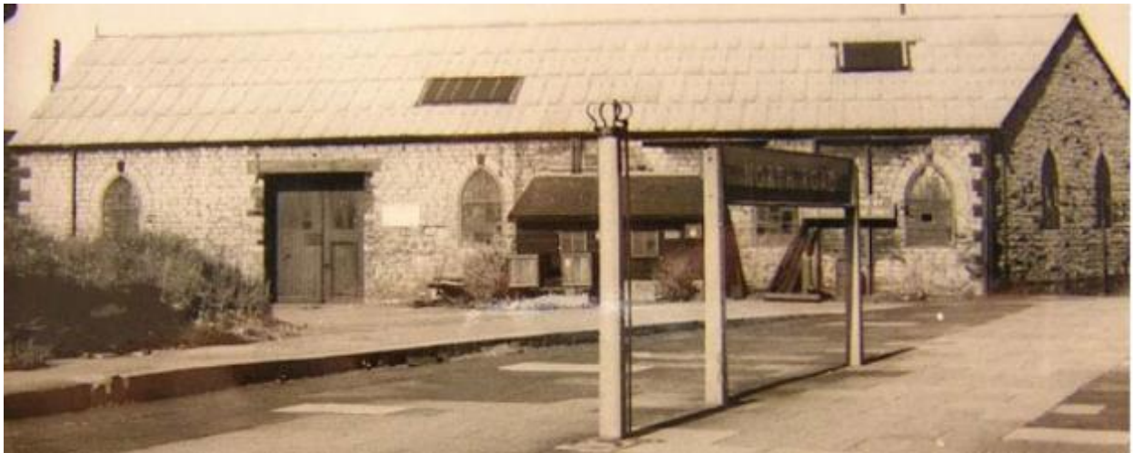
Figure 76. Kitching's foundry building remains c.1969 [taken from fig 50 in University of York CMP 2004]
