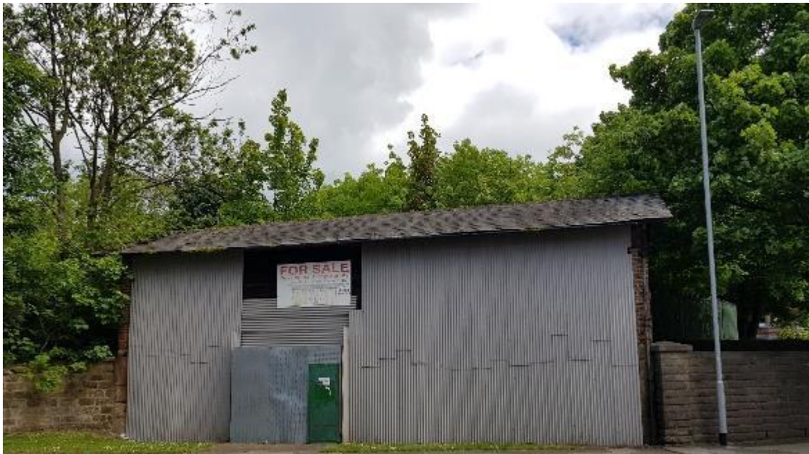
Figure 56. The lime depot. It is currently difficult to appreciate the aesthetics of its design, but it is due to be restored and a new use found before 2025
