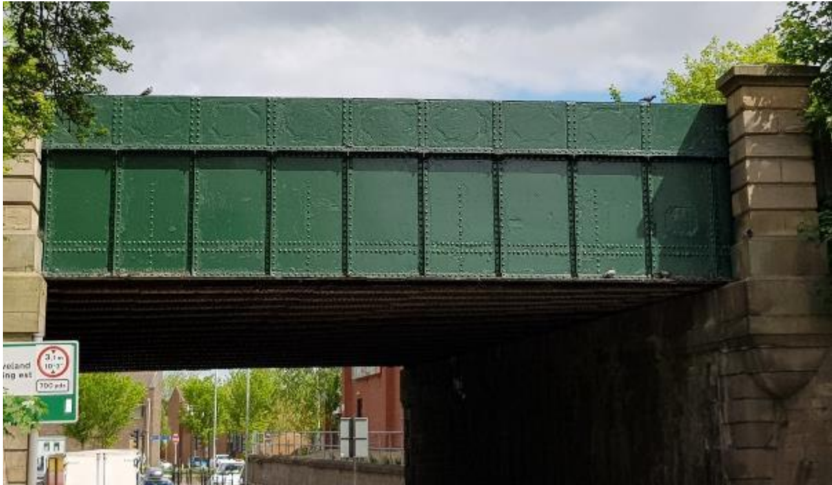
Figure 36. The replacement parapet with lozenge shapes in the top panels.
