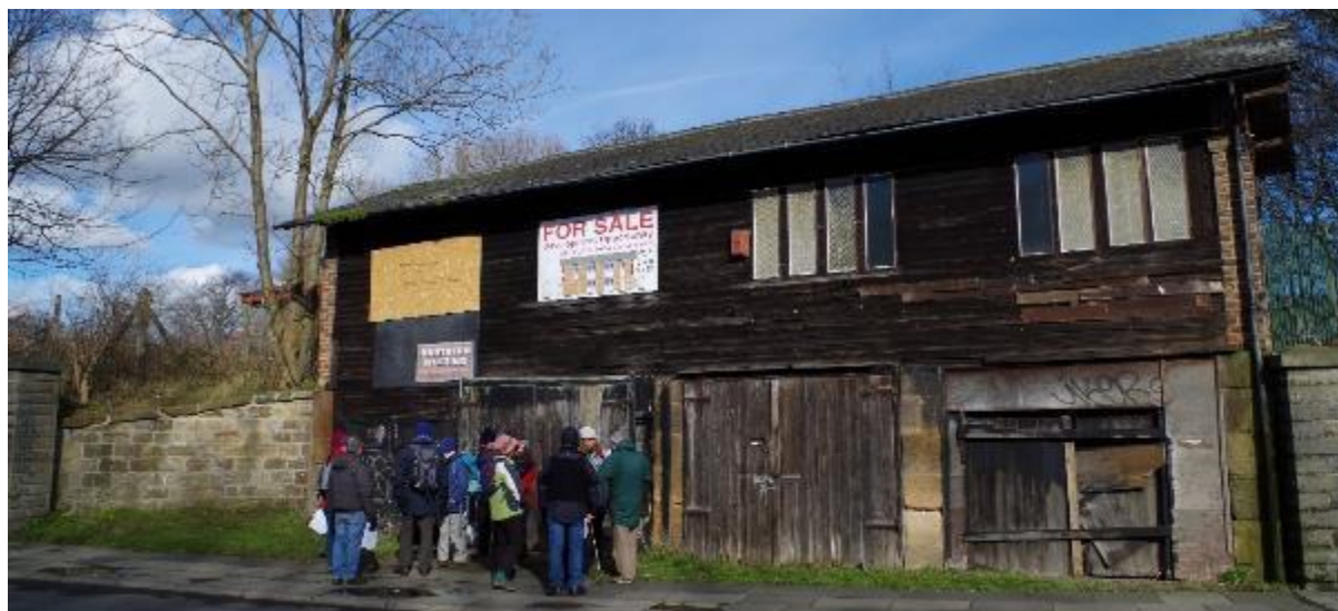
Figure 86. The lime depot being visited by the Friends of the S&DR prior to being secured behind security shuttling
