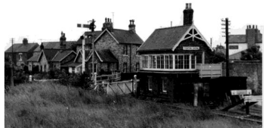
17 General view of the former crossing
