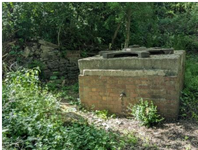
16 The crane base and ramp
