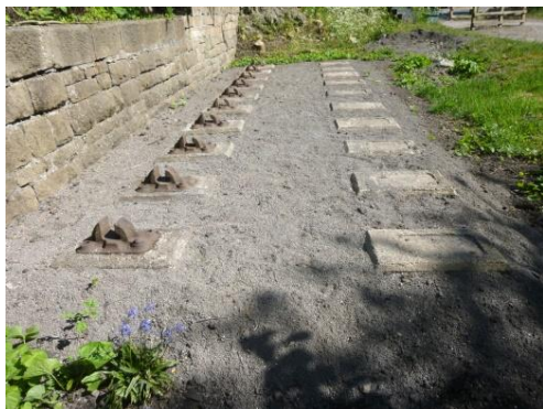
8 The track installation
