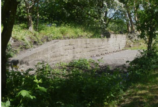
12 The Loading Dock wall in 2025
